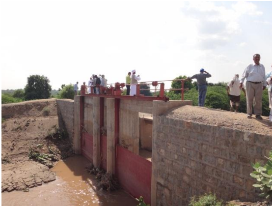
Photos (35 to 36) Improved control and off-take structure in Wadi Zabid main canal
