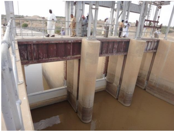
Photos (17 to 20) Wadi Mawr diversion structure, sluice gate, intakes
