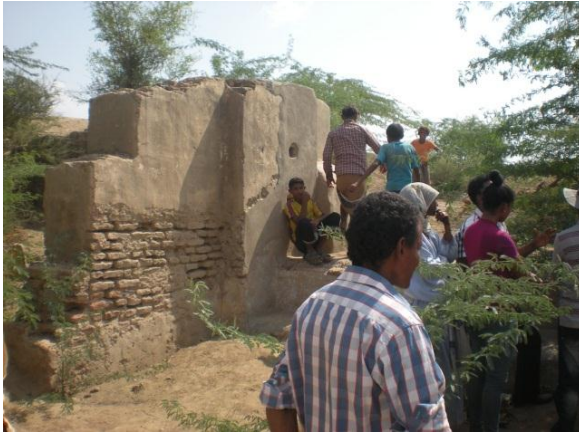
Photos (35 to 36) Traditional field spill way in Wadi Zabid irrigated fields
